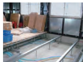
Using integrated lumber girders and floor panels
