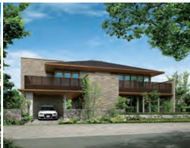
Gravis Villa SHAWOOD wooden-frame detached house
