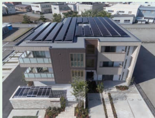
Japan's first rental housing complex where all units are ZEH (Kanazawa City, Ishikawa Prefecture)
