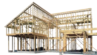
SHAWOOD construction method
