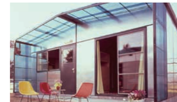
In an era when wood frame homes were the standard, the Model A homes that we built using steel, aluminum and plastic as building materials were the cutting-edge houses of the time
