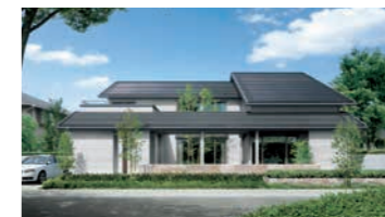
Green First Zero, a net zero energy house that provides comfortable living while reducing CO 2 emissions through the use of photovoltaic power generation
