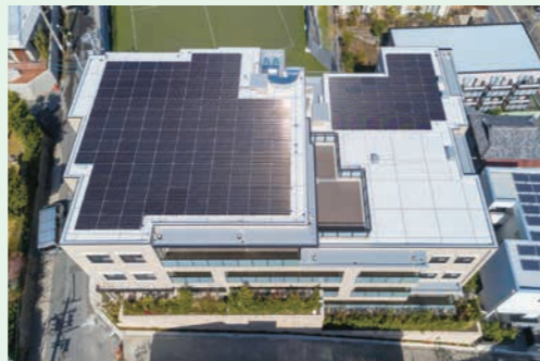
Japan's first condominium building where all units are ZEH (Nagoya City, Aichi Prefecture)
