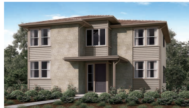
ZNE housing in California
