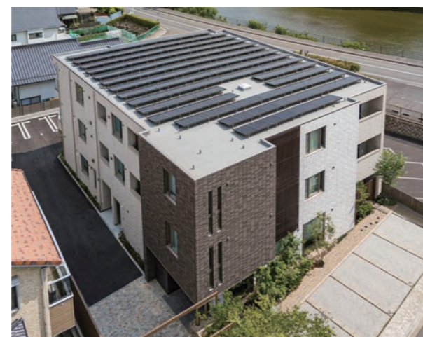
Sha Maison ZEH rental housing in Hiroshima (All units are ZEH.)
