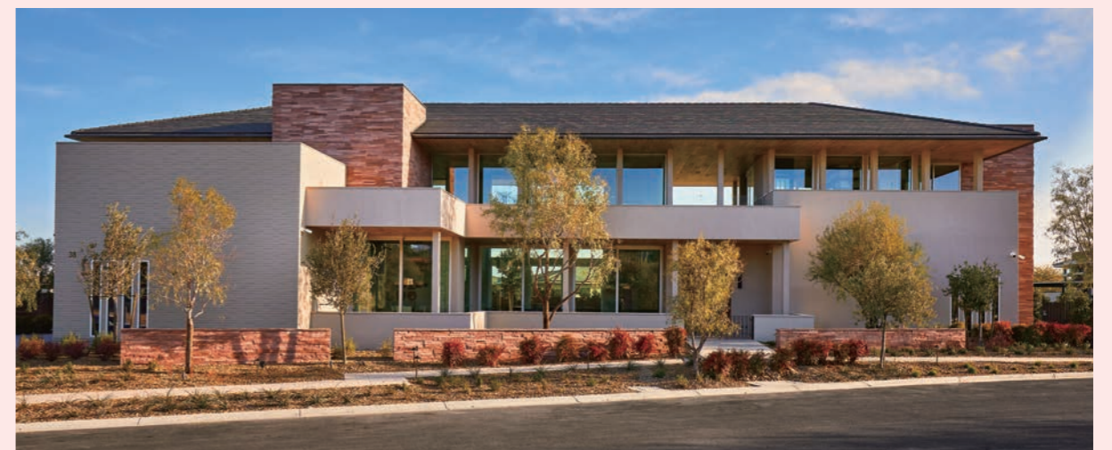
Concept home constructed in the Summerlin area of western Las Vegas
