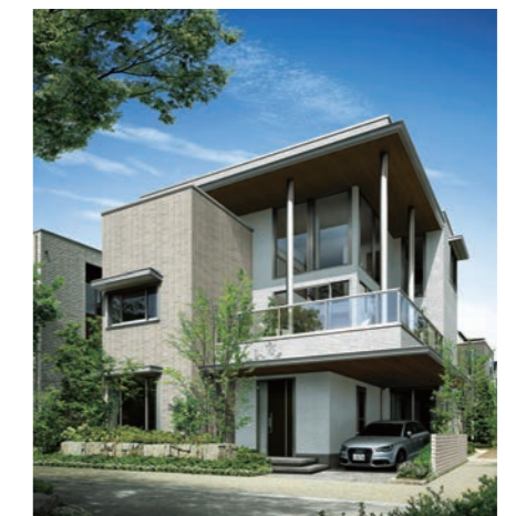
Both the open balcony space and the installation of high-capacity solar panels are made possible with columns that support the large roof on the second floor.
