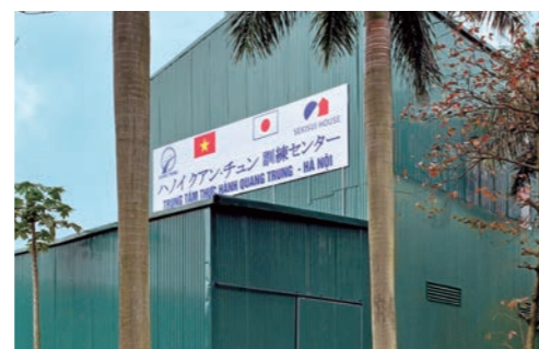
Technical training center in Hanoi, Vietnam (exterior)
