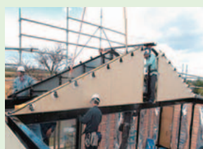
Installing a precut piece of plasterboard as boundary wall for an attic
