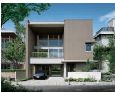
Biena three-story steel-frame detached house
