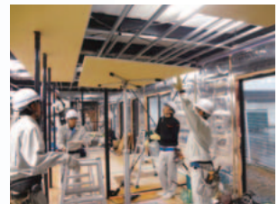
On-site training for installing plasterboard on ceilings
