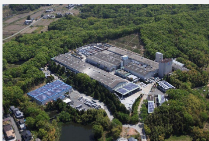
Hyogo Factory mega solar
