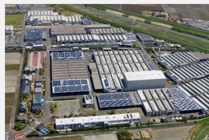
Shizuoka Factory mega solar
