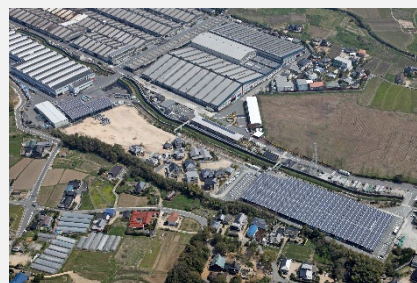
Yamaguchi Factory mega solar
