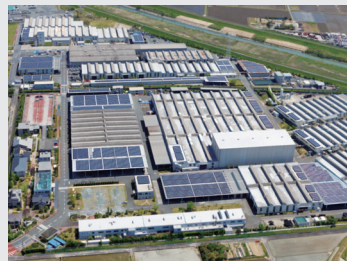
Shizuoka Factory mega solar
