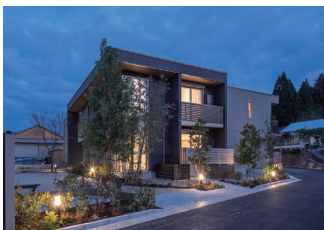
Exterior of Promoting Permanent Residency Housing in Yamato Town, Kumamoto Prefecture
