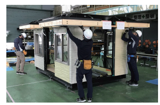
Framing/exterior course: completion test
