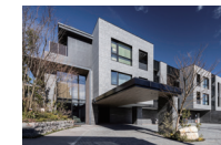
Mejirozaka Terrace: Low-rise housing created in harmony with the tranquil residential area
