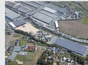
Yamaguchi Factory mega solar
