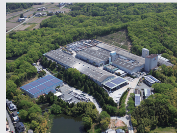
Hyogo Factory mega solar
