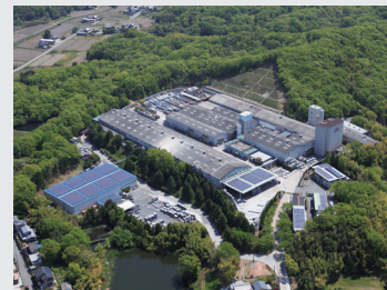
Hyogo Factory mega solar
