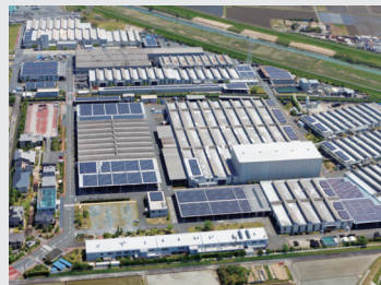
Shizuoka Factory mega solar
